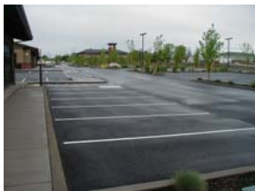
Exceptional grading design keeps parking lots dry even during the heaviest storms
